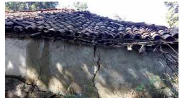
A cracked mud wall of a house
